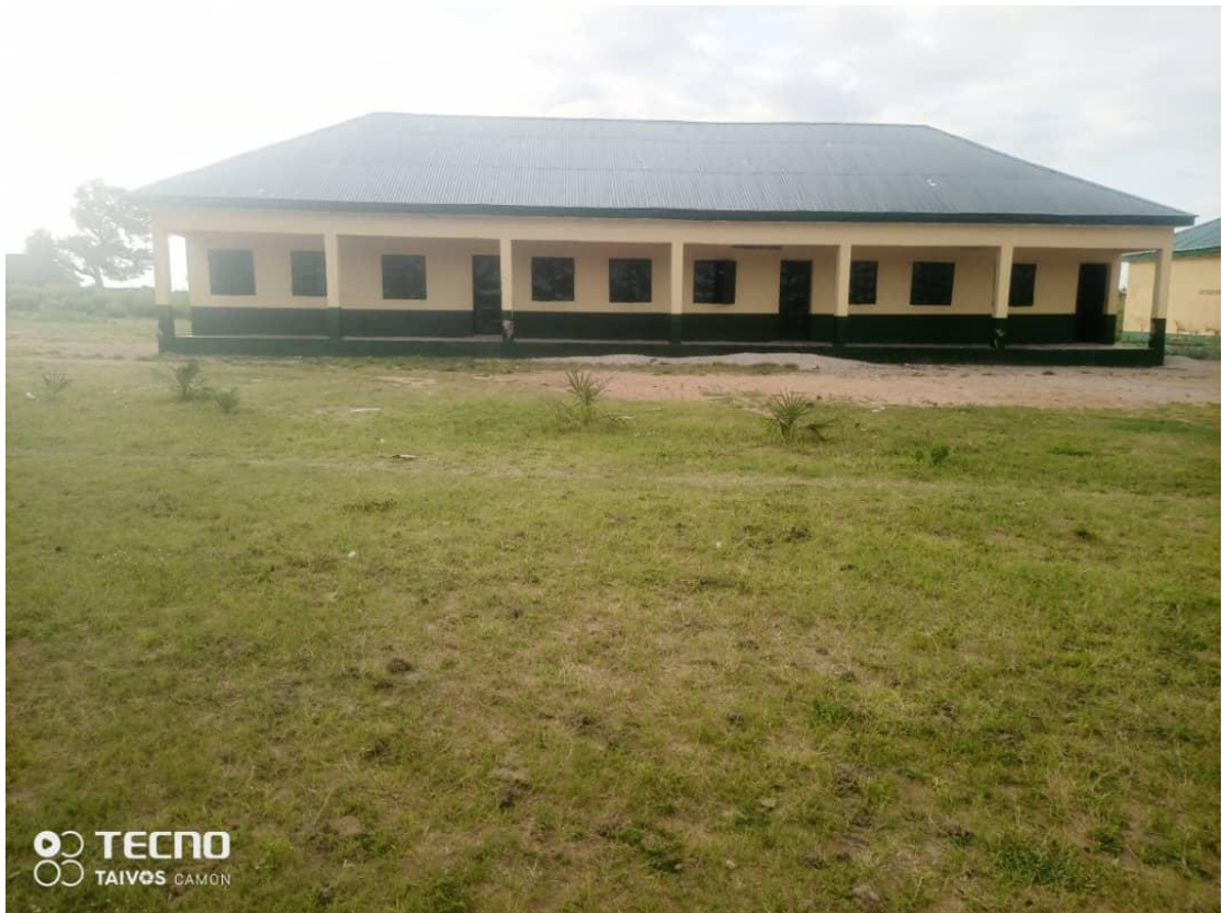
REHABILITATION OF A BLOCK OF 3 CLASSROOMS OFFICE AND STORE AT APPAWA SHANGAL PRIMARY SCHOOL IN LAU L.G.A(BEFORE AND AFTER)
