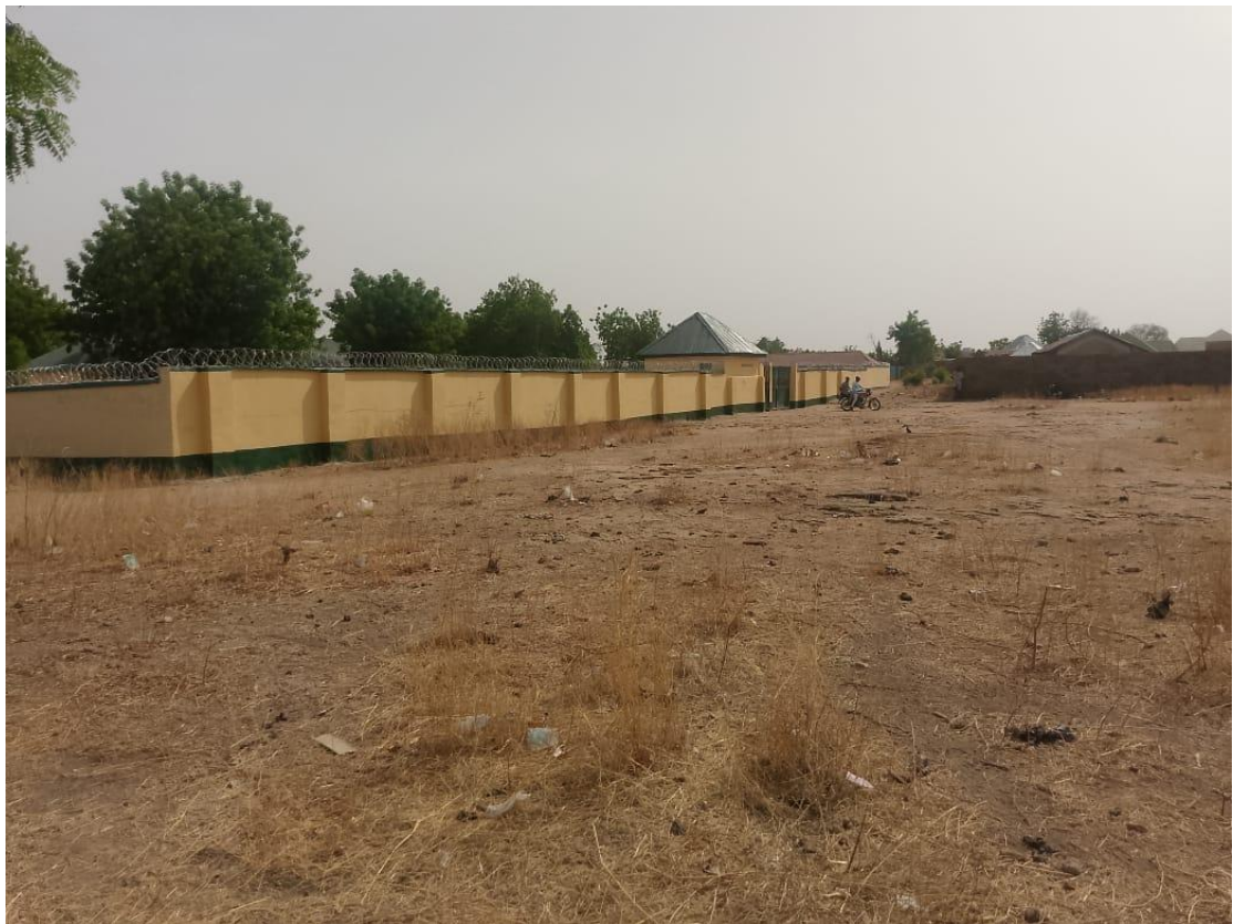
CONSTRUCTION OF A PEREMETER FENCE WALL AT SAYONTI PRIMARY SCHOOL IN LAU L.G.A
