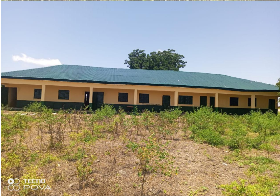
REHABILITATION OF A BLOCK OF 3 CLASSROOMS OFFICE AND STORE AT KARIM WEST PRIMARY SCHOOL KARIM LAMIDO L.G.A(BEFORE AND AFTER)
