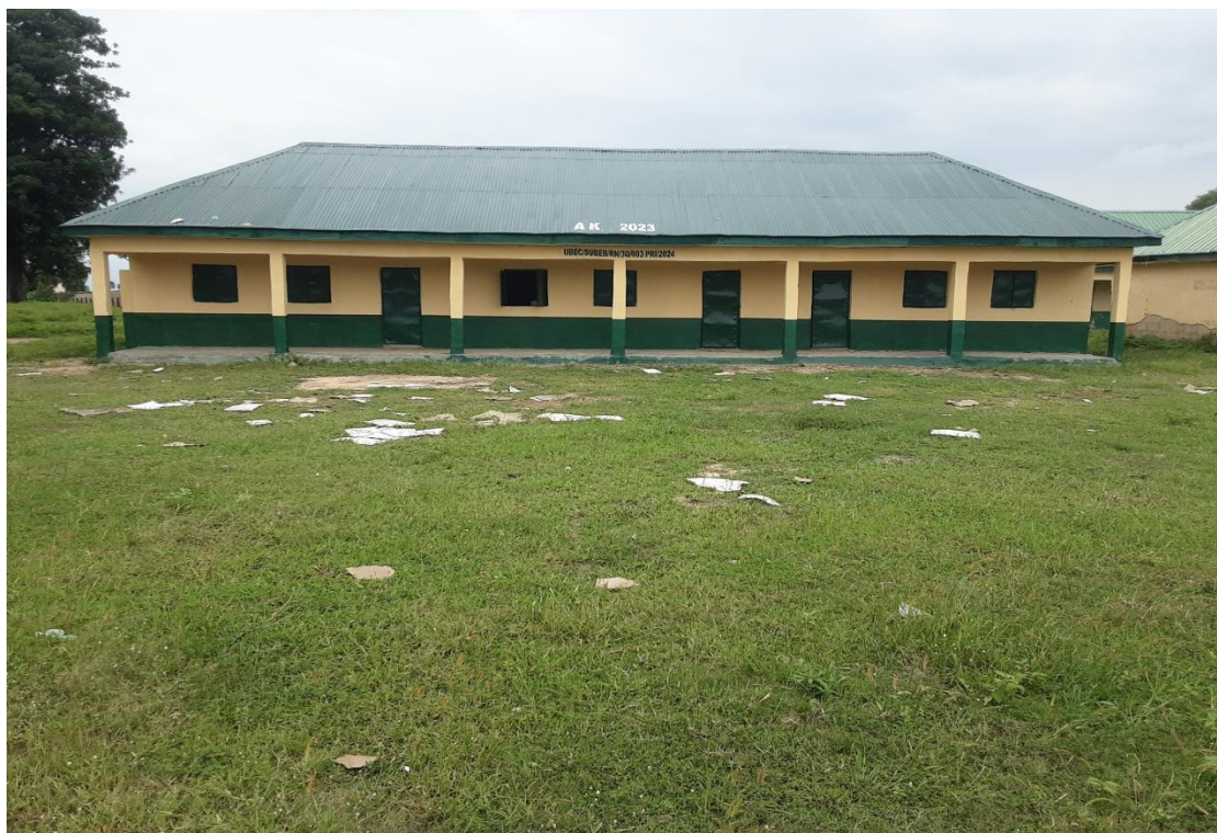
REHABILITATION OF A BLOCK OF 3 CLASSROOMS AT JENPETEL PRIMARY SCHOOL IN KARIM LAMIDO L.G.A(BEFORE AND AFTER)
