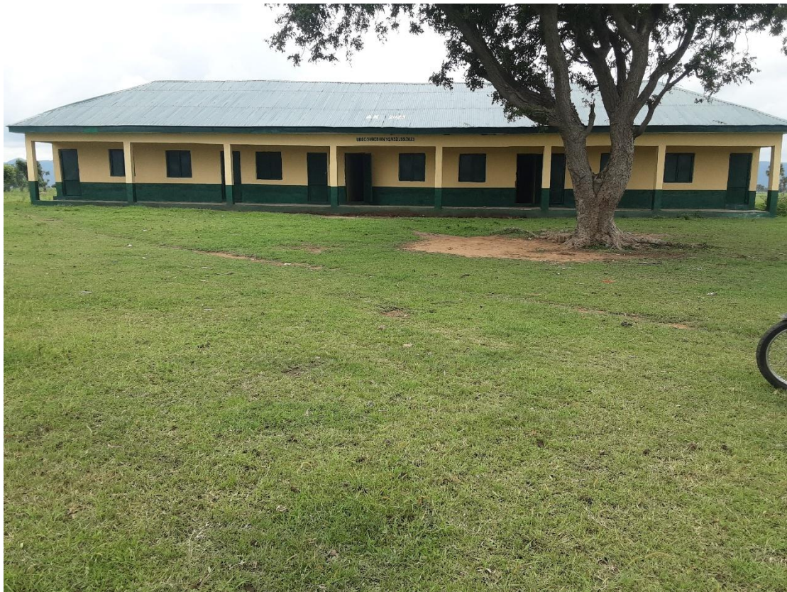
REHABILITATION OF A BLOCK OF 3 CLASSROOMS OFFICE AND STORE AT GDJSS SABONGARI IN KARIM LAMIDO L.G.A(BEFORE AND AFTER)
