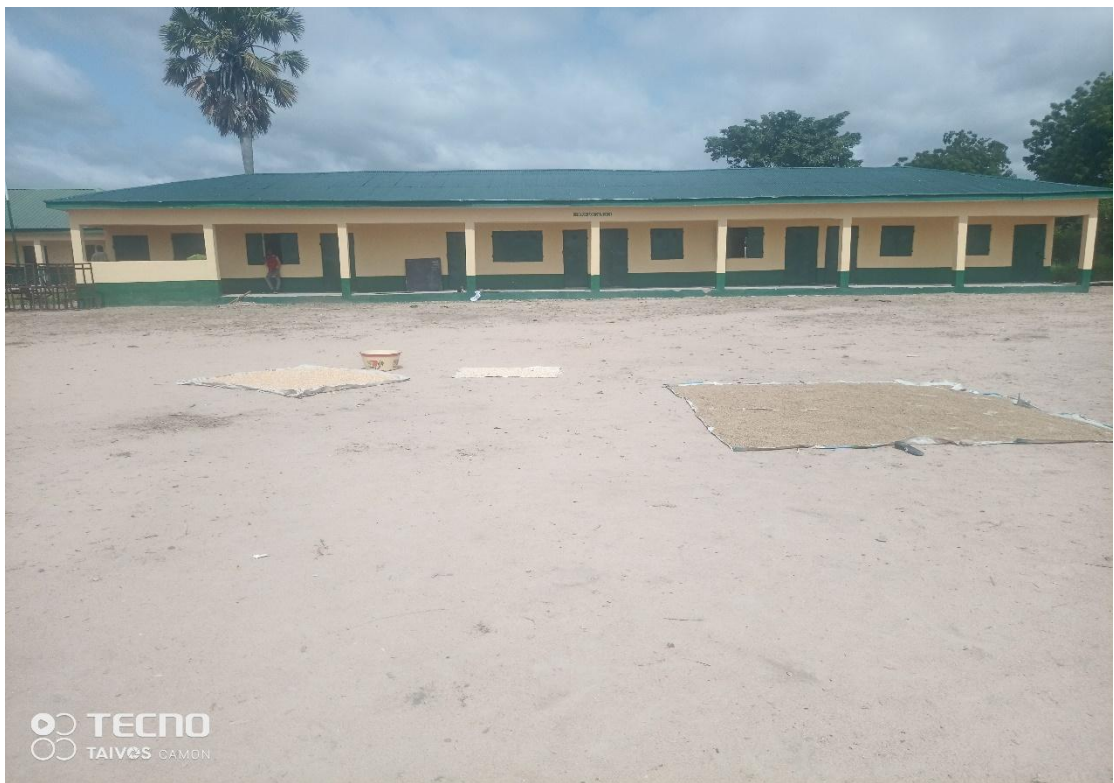
REHABILITATION OF A BLOCK OF 3 CLASSROOMS OFFICE AND STORE AT GDJSS YUSA B IN LAU L.G.A(BEFORE AND AFTER)
