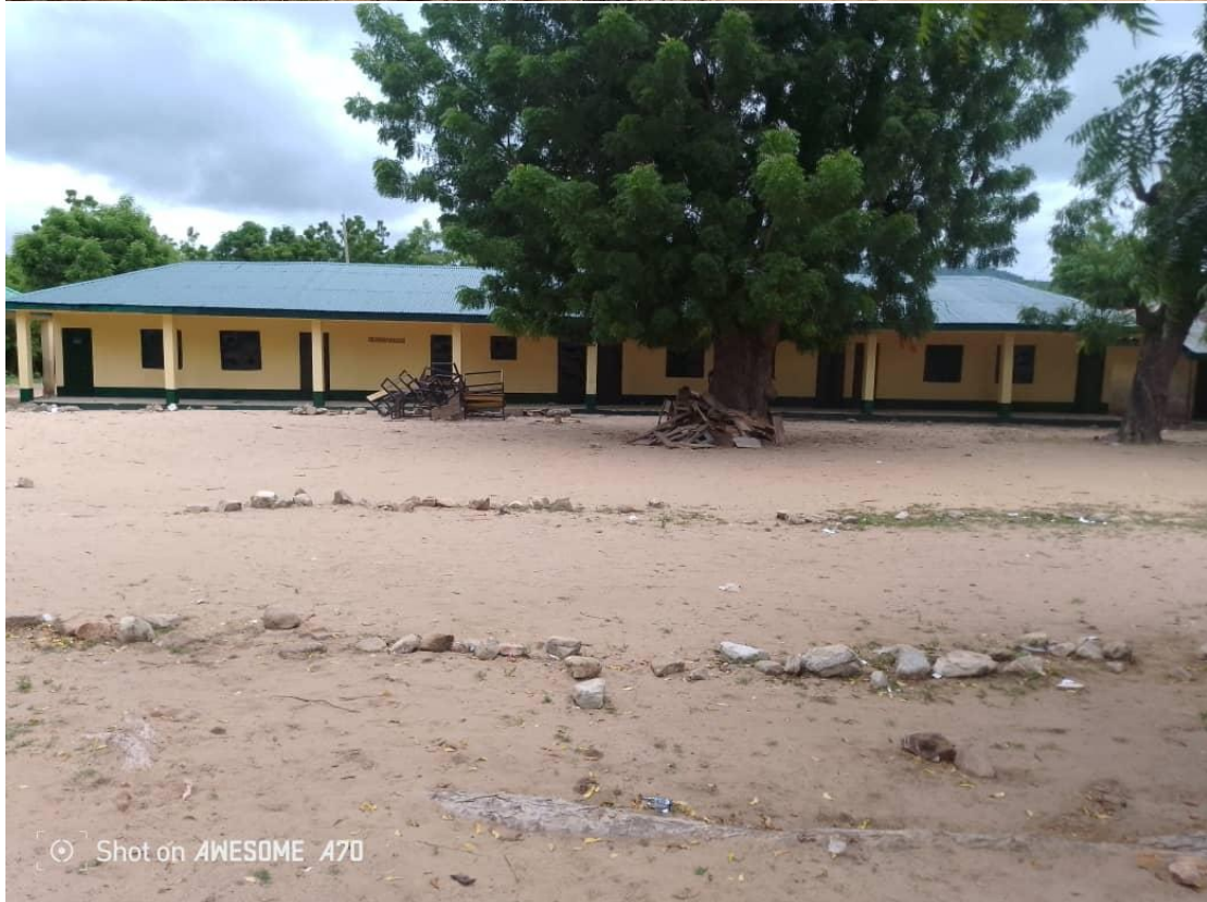
REHABILITATION OF A BLOCK OF 3 CLASSROOMS OFFICE AND STORE AT GDJSS MUTUM DAYA IN KARIM LAMIDO L.G.A(BEFORE AND AFTER)
