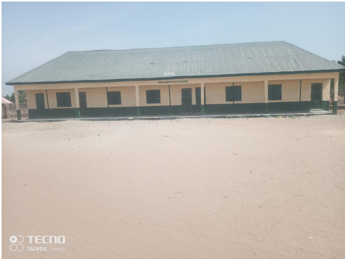
REHABILITATION OF A BLOCK OF 2 CLASSROOMS OFFICE AND STORE AT GJTTS IN KARIM LAMIDO L.G.A(BEFORE AND AFTER)
