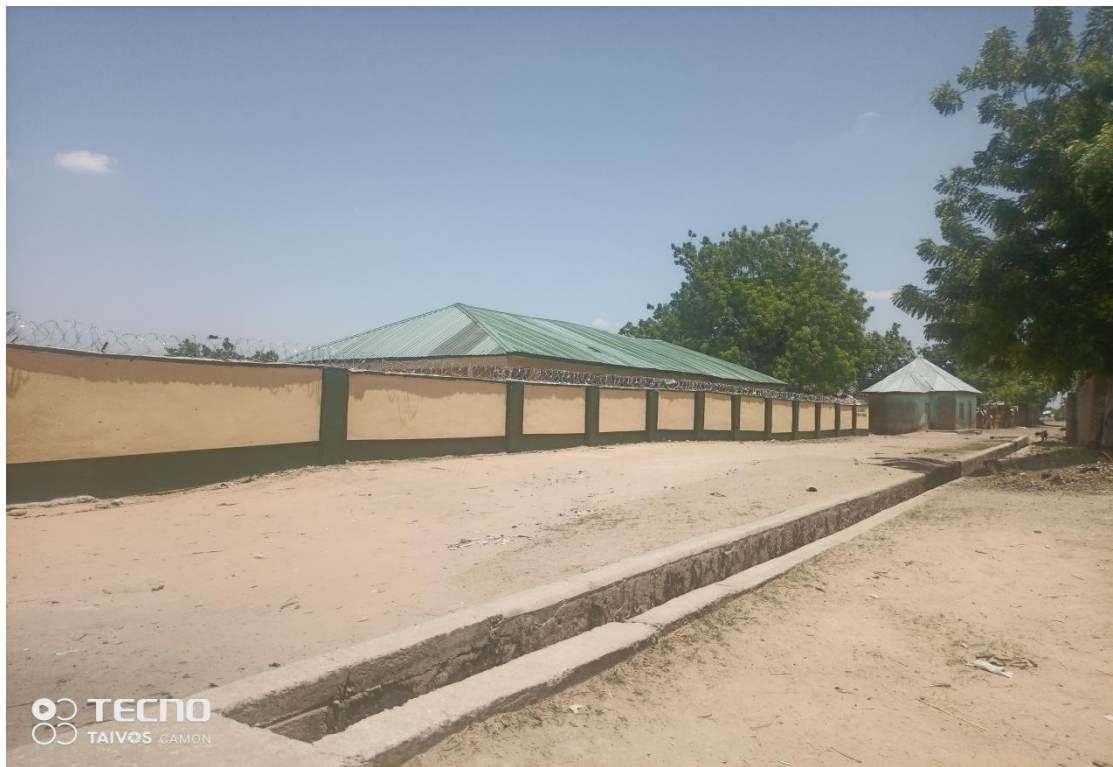
CONSTRUCTION OF A PEREMETER FENCE WALL AT KARIM CENTRAL PRIMARY SCHOOL IN KARIM LAMIDO L.G.A
