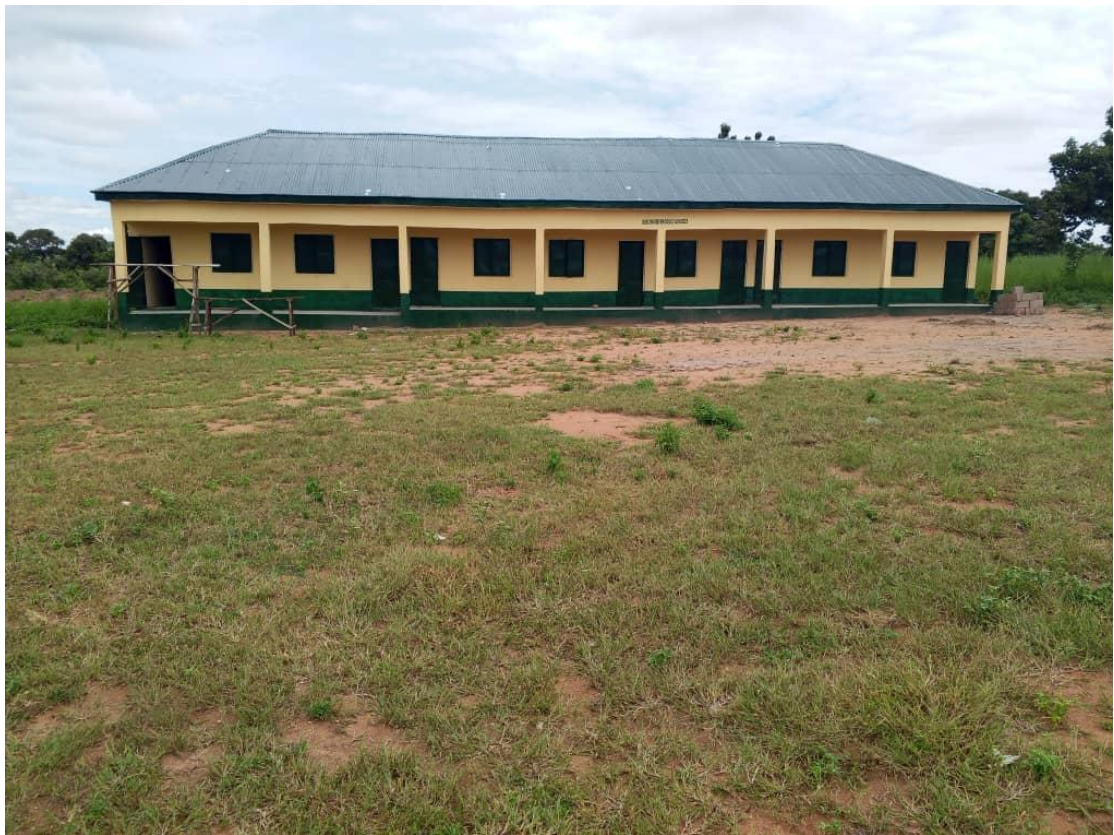
REHABILITATION OF A BLOCK OF 3 CLASSROOMS OFFICE AND STORE AT APPAWA LUBE PRIMARY SCHOOL IN LAU L.G.A(BEFORE AND AFTER)
