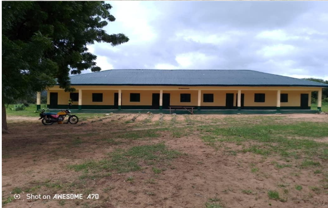
REHABILITATION OF A BLOCK OF 3 CLASSROOMS OFFICE AND STORE AT GANGAN BALASA PRIMARY SCHOOL IN KARIM LAMIDO L.G.A(BEFORE AND AFTER)
