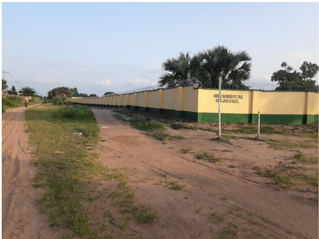
CONSTRUCTION OF A PEREMETER FENCE WALL AT GARIN DOGO PRIMARY SCHOOL IN LAU L.G.A
