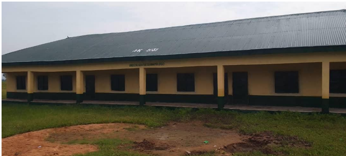
REHABILITATION OF A BLOCK OF 3 CLASSROOMS OFFICE AND STORE AT MUNGA LELAU PRIMARY SCHOOL IN KARIM LAMIDO L.G.A(BEFORE AND AFTER)
