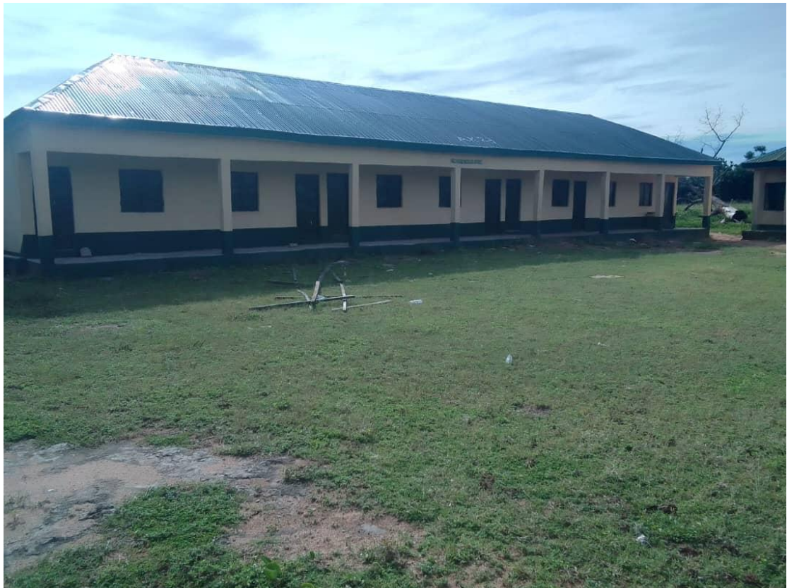
REHABILITATION OF A BLOCK OF 3 CLASSROOMS OFFICE AND STORE AT GDJSS ABBARE IN LAU L.G.A(BEFORE AND AFTER)
