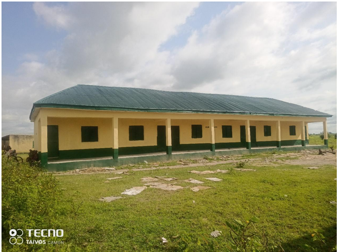
REHABILITATION OF A BLOCK OF 3 CLASSROOMS OFFICE AND STORE AT GDJSS KUNINI IN LAU L.G.A(BEFORE AND AFTER)
