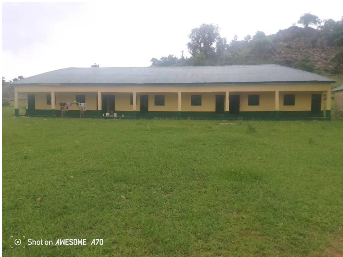
REHABILITATION OF A BLOCK OF 3 CLASSROOMS OFFICE AND STORE AT PIRIBI PRIMARY SCHOOL IN KARIM LAMIDO L.G.A(BEFORE AND AFTER)
