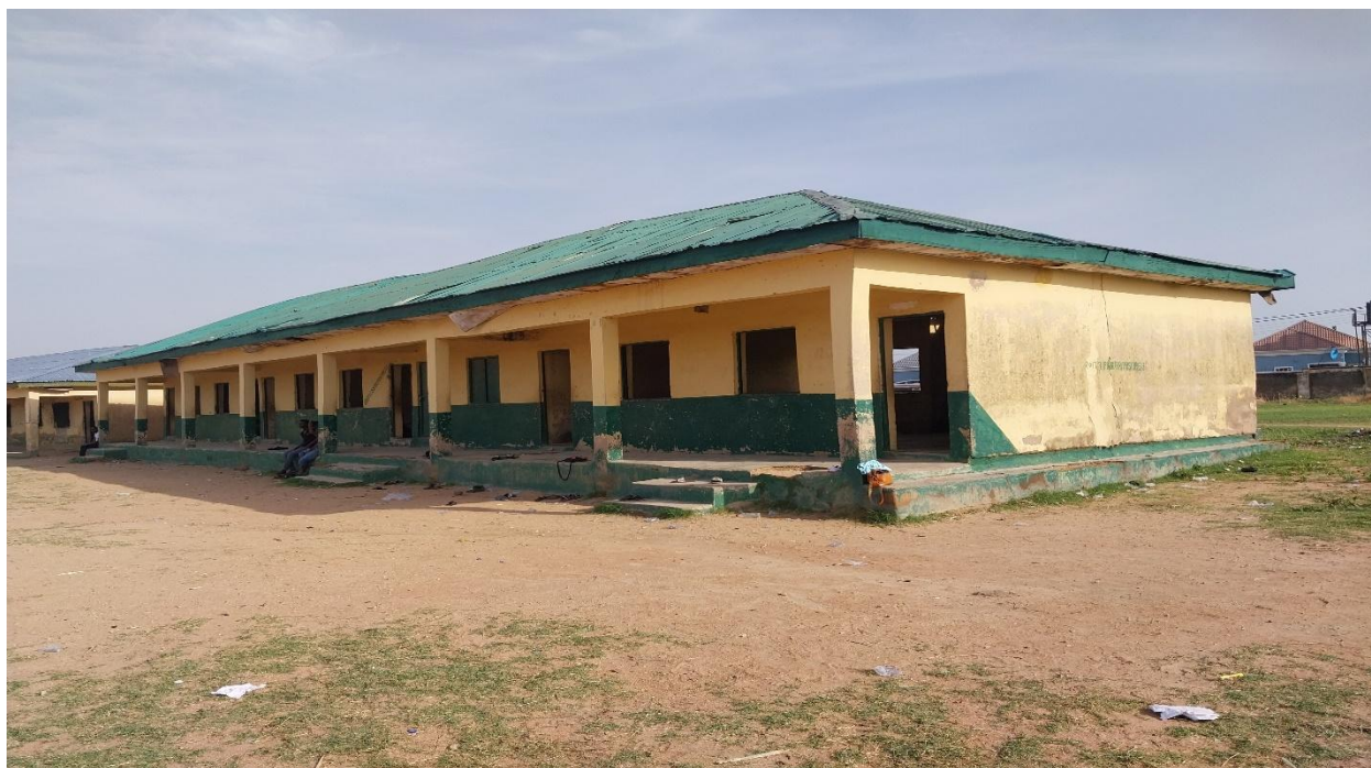
SALIHU DOGO PRIMARY SCHOOL JALINGO- BLOCK B, 3 CLASSROOMS, OFFICE AND STORE (BEFORE)
