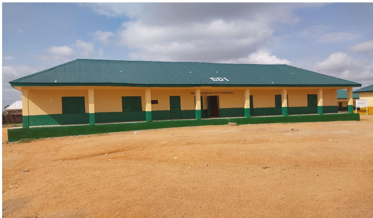
MOH'D TUKUR PRIMARY SCHOOL JALINGO- BLOCK A, 2 CLASSROOMS, OFFICE AND STORE (AFTER)
