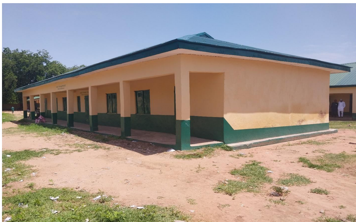
HASSAN PRIMARY SCHOOL JALINGO- BLOCK A, 2 CLASSROOMS, OFFICE AND STORE (AFTER)
