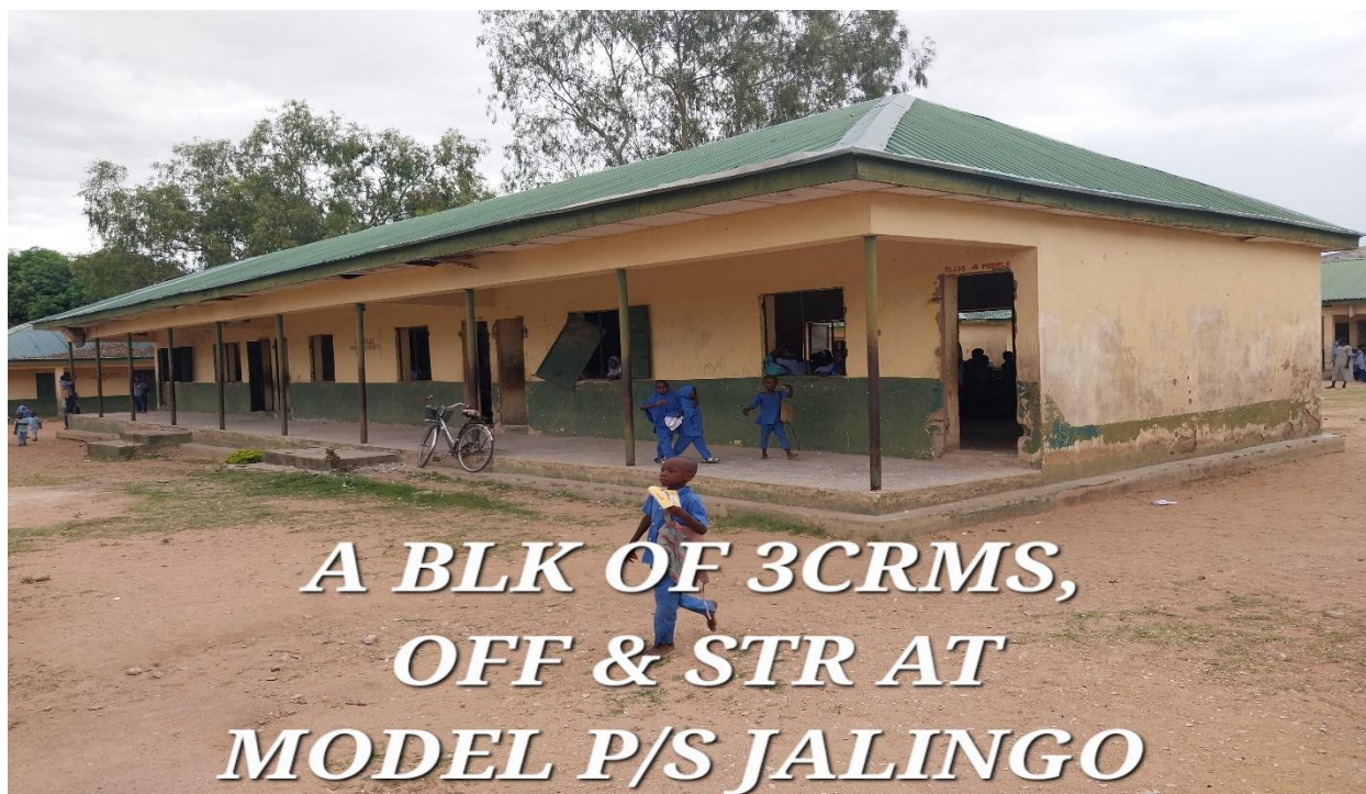
MODEL PRIMARY SCHOOL JALINGO- BLOCK A, 3 CLASSROOMS, OFFICE AND STORE (BEFORE)
