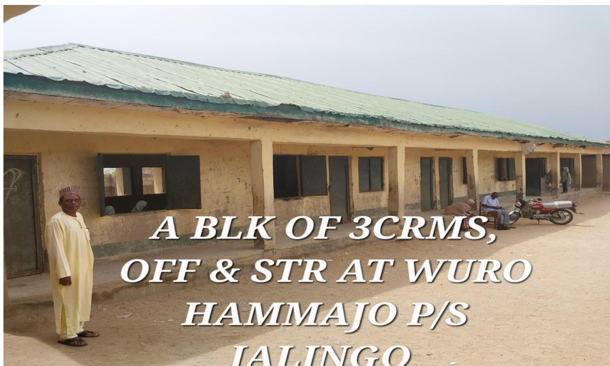
WURO HAMMAJO PRIMARY SCHOOL JALINGO- BLOCK A, 3 CLASSROOMS, OFFICE AND STORE (BEFORE)
