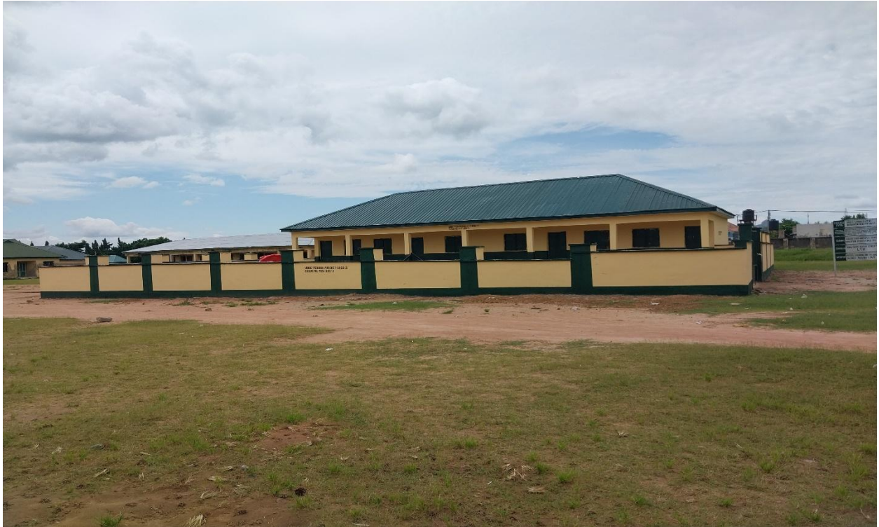
SALIHU DOGO PRIMARY SCHOOL JALINGO- CONSTRUCTION OF A BLOCK OF 2 CLASSROOMS, OFFICES, INTERNAL TOILET AND DWARF FENCE
