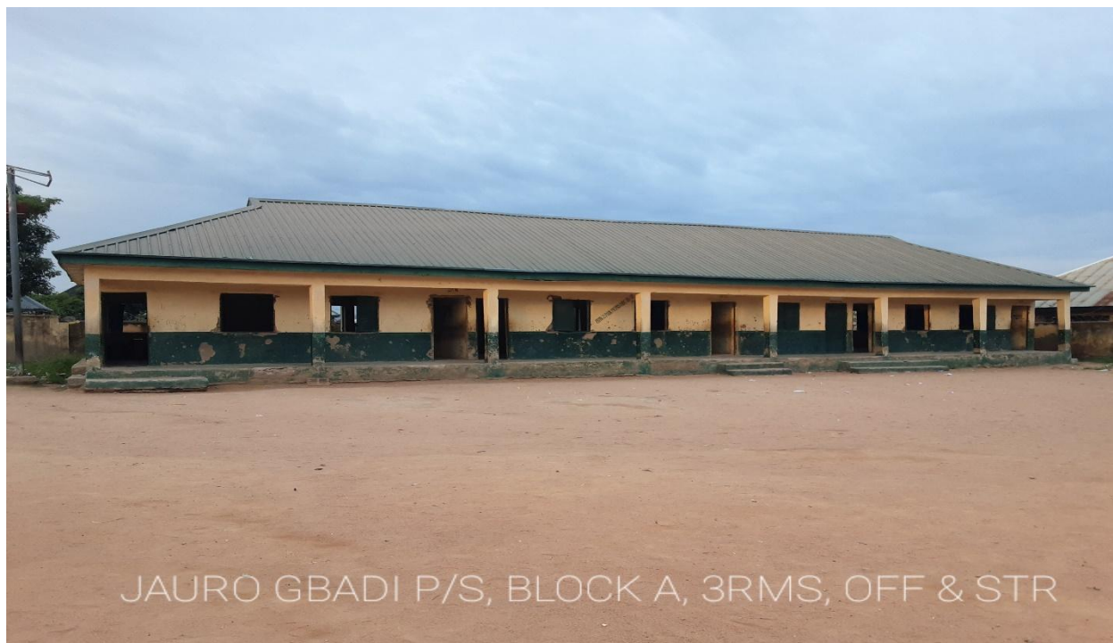
JAURO GBADI PRIMARY SCHOOL JALINGO- BLOCK A, 3 CLASSROOMS, OFFICE AND STORE (BEFORE)
