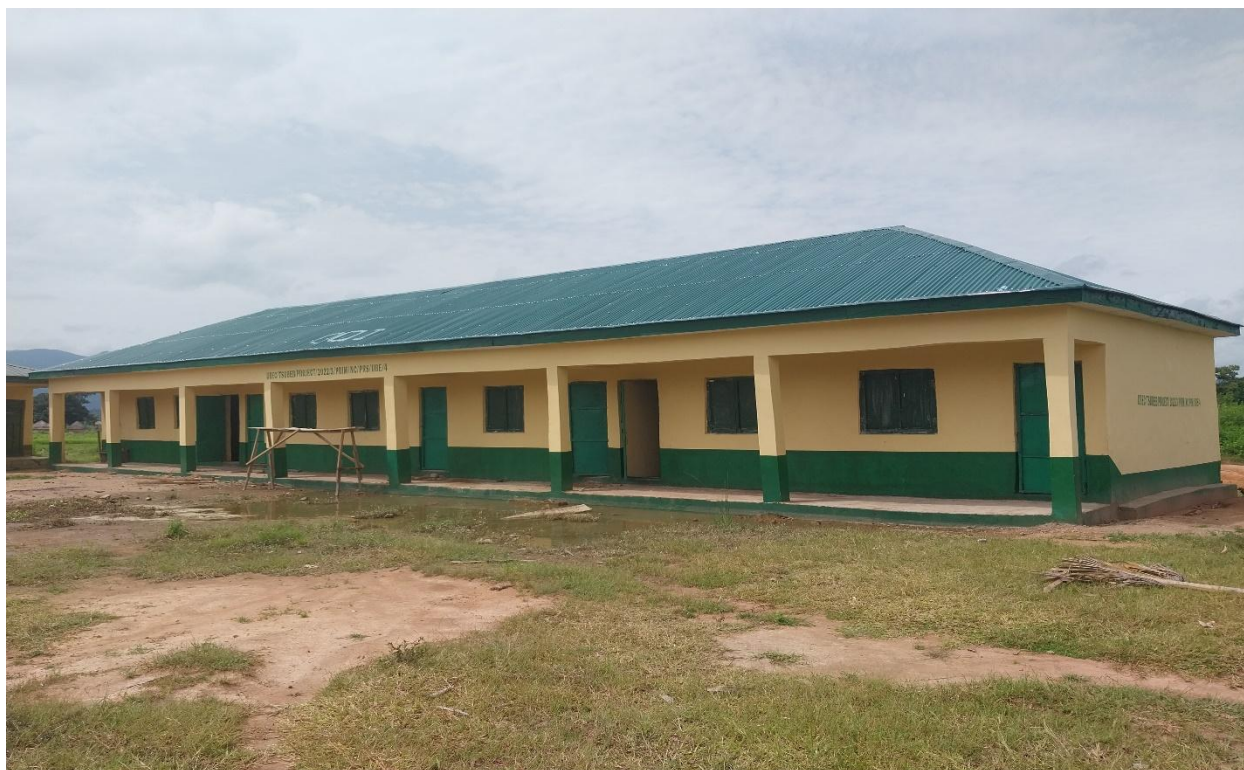
GONGON MAIHUJJA PRIMARY SCHOOL JALINGO- CONSTRUCTION OF A BLOCK OF 3 CLASSROOMS, OFFICE AND STORE
