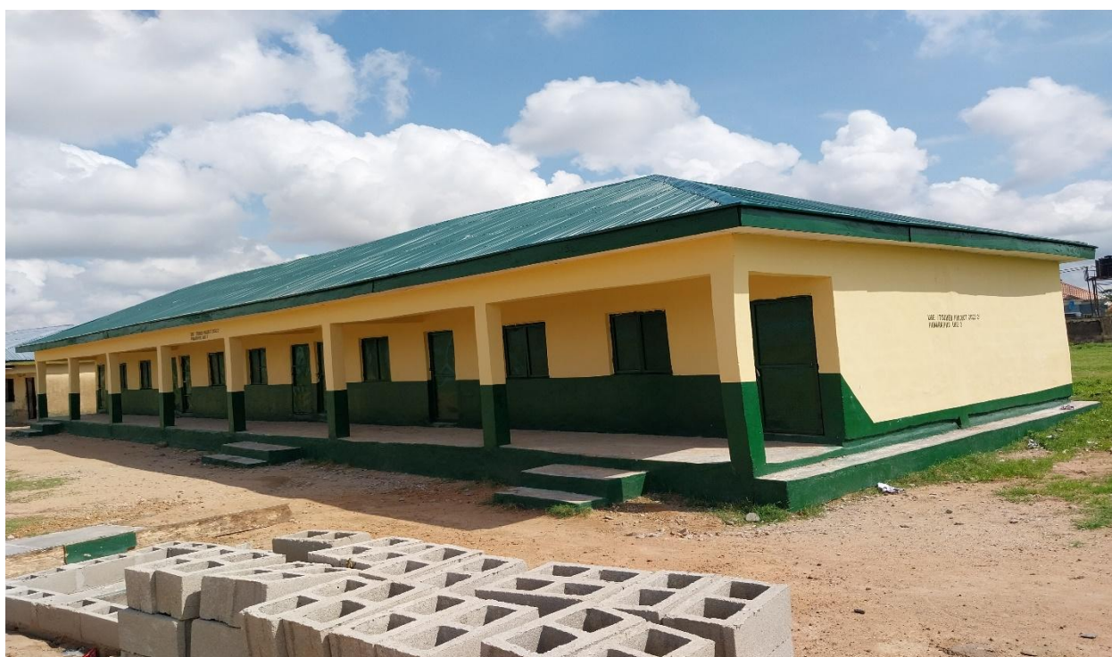
SALIHU DOGO PRIMARY SCHOOL JALINGO- BLOCK B, 3 CLASSROOMS, OFFICE AND STORE (AFTER)
