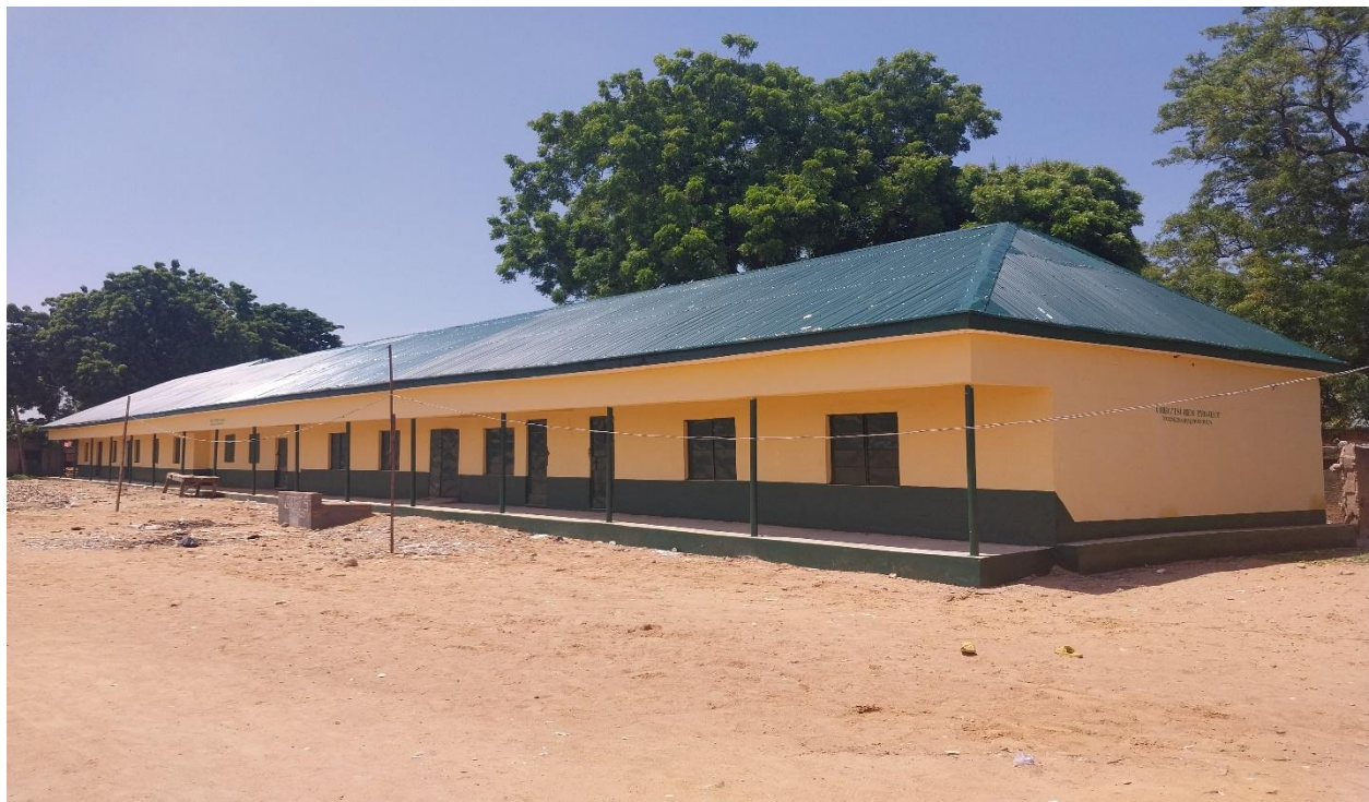
GOVERNMENT JUNIOR TECHNICAL COLLEGE JALINGO- BLOCK A, 6 CLASSROOMS, OFFICE AND STORE (AFTER)
