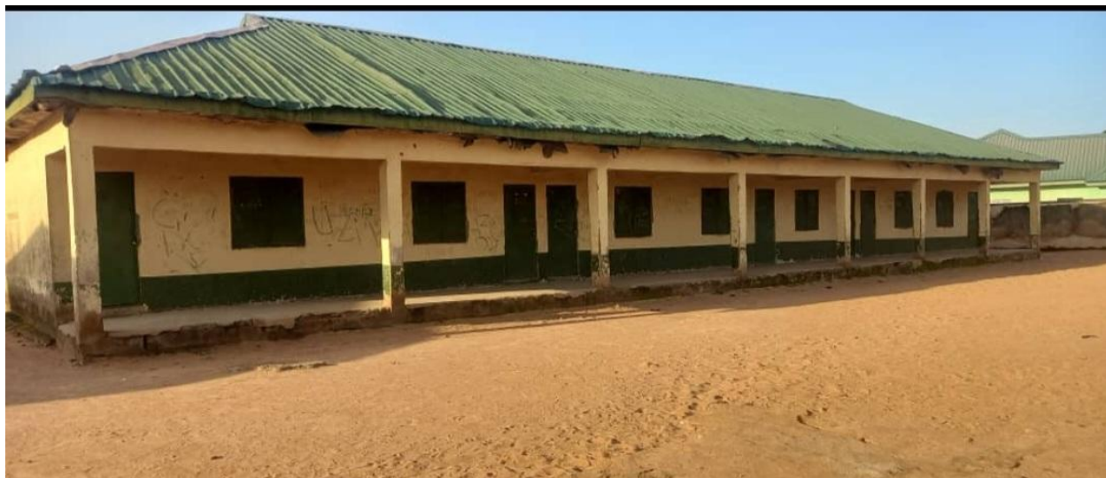
MAFINDI PRIMARY SCHOOL JALINGO- BLOCK A, 3 CLASSROOMS, OFFICE AND STORE(BEFORE)
