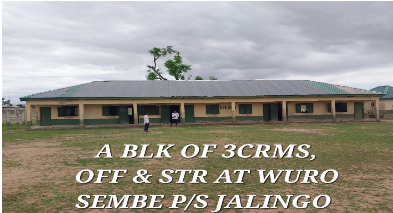
WURO SEMBE PRIMARY SCHOOL JALINGO- BLOCK B, 3 CLASSROOMS, OFFICE AND STORE (BEFORE)
