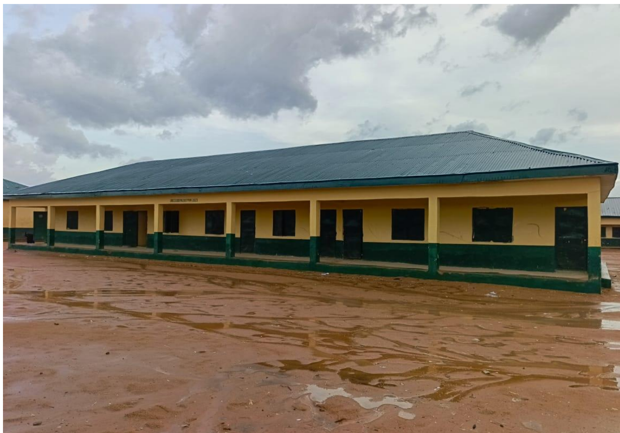
MAFINDI PRIMARY SCHOOL JALINGO- BLOCK A, 3 CLASSROOMS, OFFICE AND STORE (AFTER)
