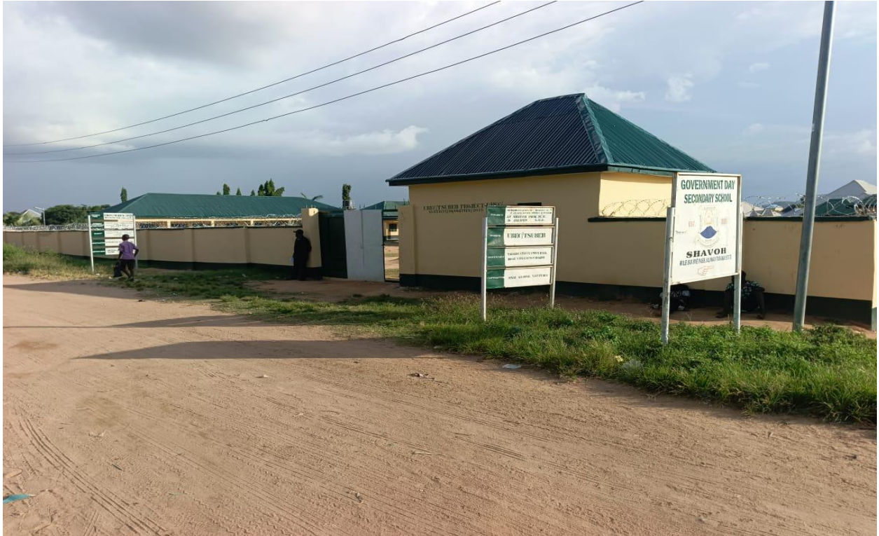
SHAVOH PRIMARY SCHOOL- CONSTRUCTION OF PERIMETER FENCE WALL
