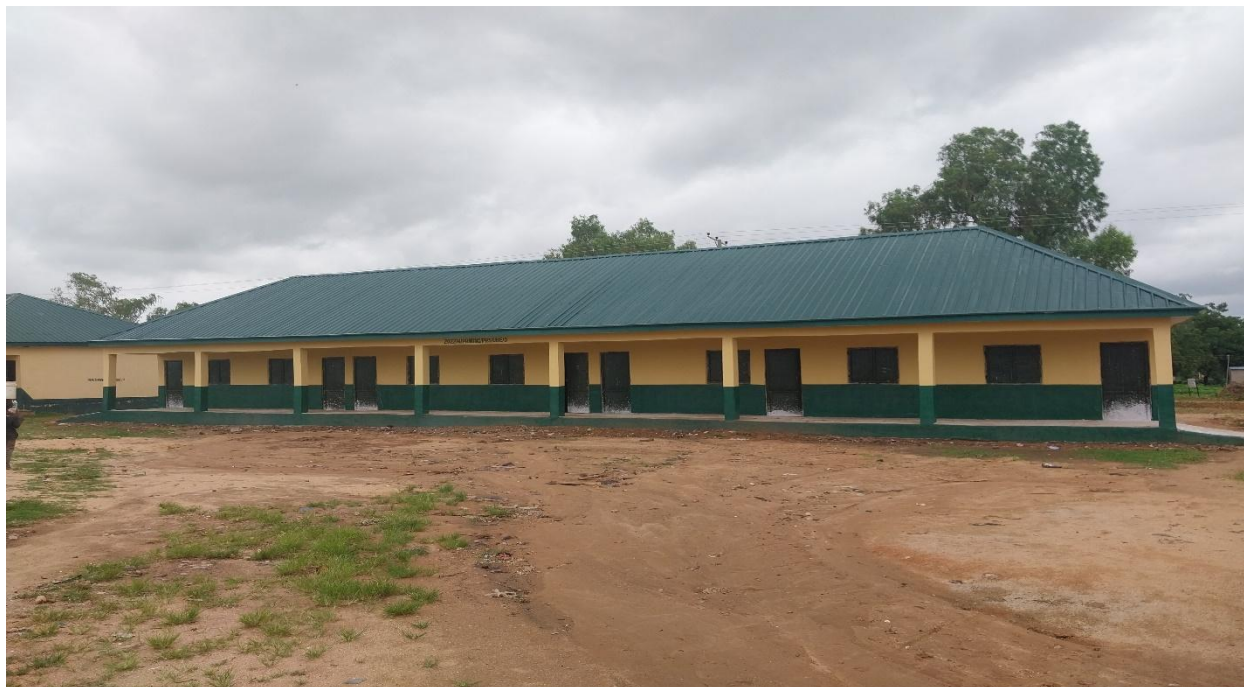
ADULT AND LITERACY CENTER JALINGO- CONSTRUCTION OF A BLOCK OF 3 CLASSROOMS, OFFICE AND STORE
