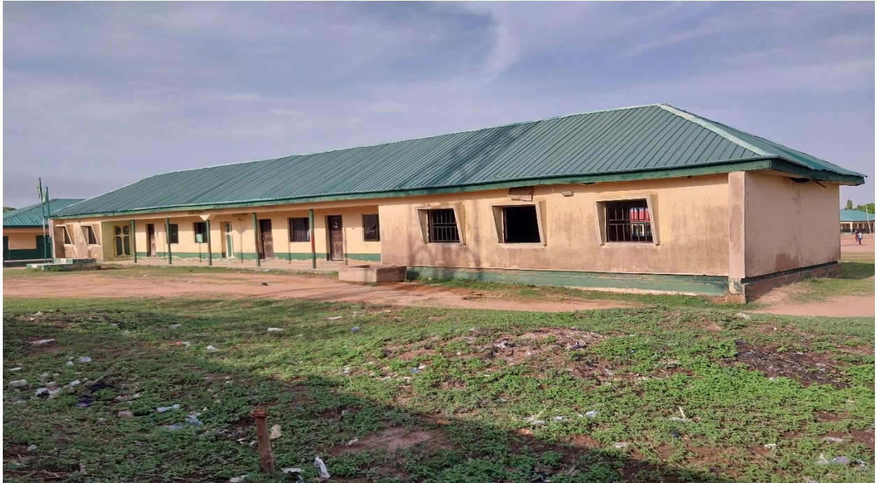
SALIHU DOGO PRIMARY SCHOOL JALINGO- BLOCK A, 3 CLASSROOMS, OFFICE AND STORE (BEFORE)
