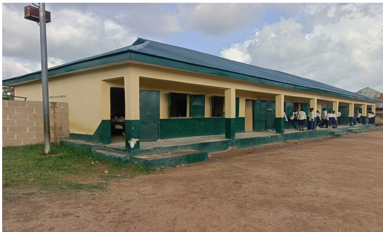
JAURO GBADI PRIMARY SCHOOL JALINGO- BLOCK A, 3 CLASSROOMS, OFFICE AND STORE (AFTER)
