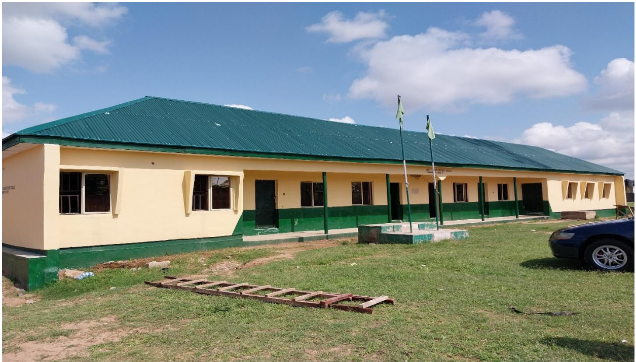
SALIHU DOGO PRIMARY SCHOOL JALINGO- BLOCK A, 3 CLASSROOMS, OFFICE AND STORE (AFTER)
