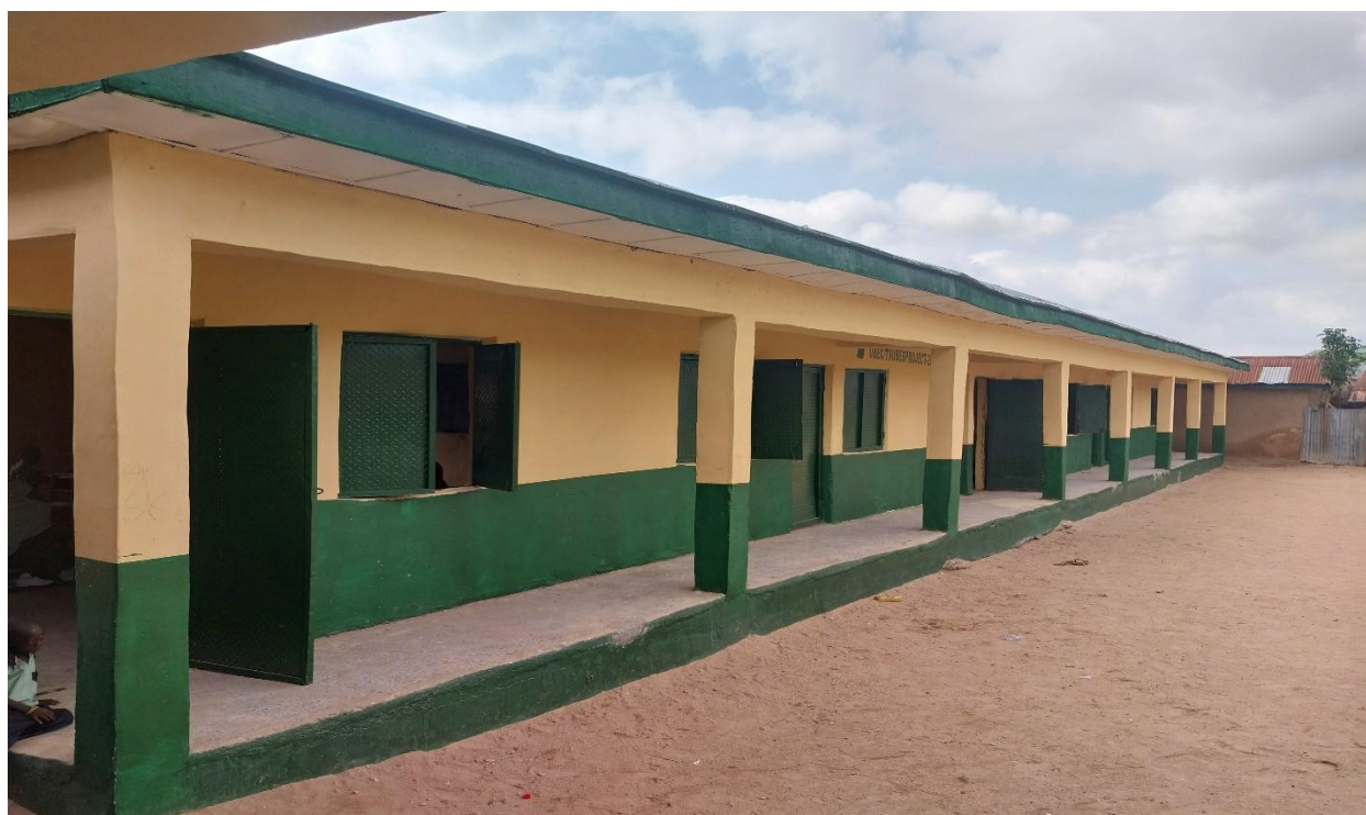
WURO HAMMAJO PRIMARY SCHOOL JALINGO- BLOCK A, 3 CLASSROOMS, OFFICE AND STORE (AFTER)
