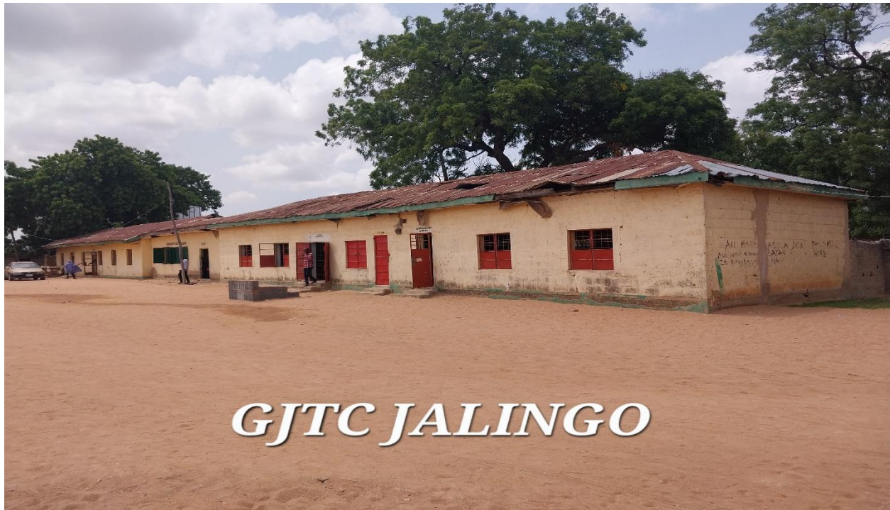
GOVERNMENT JUNIOR TECHNICAL COLLEGE JALINGO- BLOCK A, 6 CLASSROOMS, OFFICE AND STORE (BEFORE)
