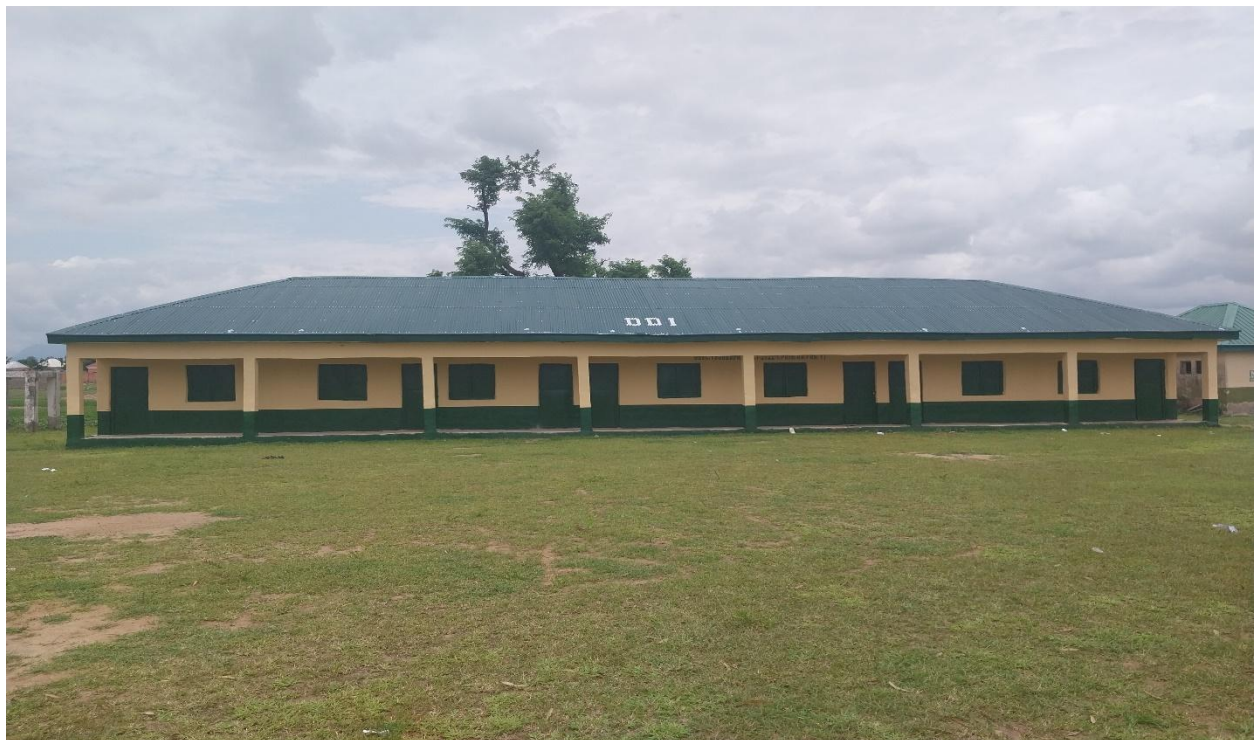
WURO SEMBE PRIMARY SCHOOL JALINGO- BLOCK B, 3 CLASSROOMS, OFFICE AND STORE (AFTER)
