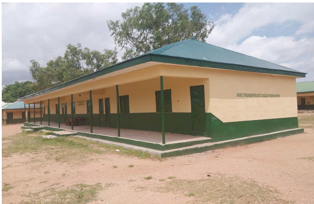
MODEL PRIMARY SCHOOL JALINGO- BLOCK A, 3 CLASSROOMS, OFFICE AND STORE (AFTER)
