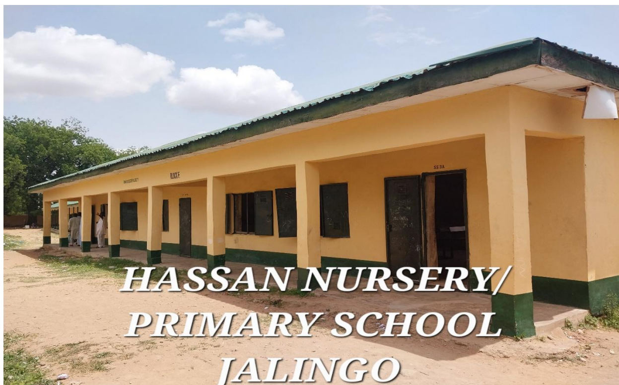
HASSAN PRIMARY SCHOOL JALINGO- BLOCK A, 2 CLASSROOMS, OFFICE AND STORE (BEFORE)
