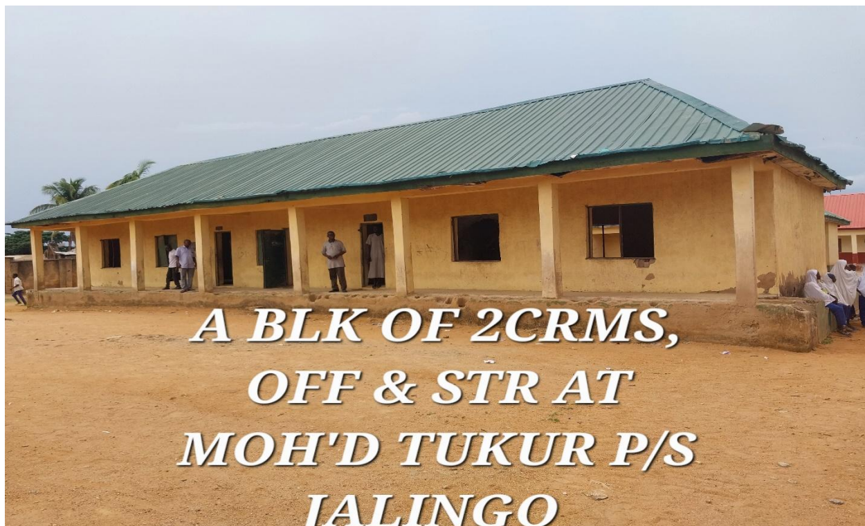
MOH'D TUKUR PRIMARY SCHOOL JALINGO- BLOCK A, 2 CLASSROOMS, OFFICE AND STORE (BEFORE)
