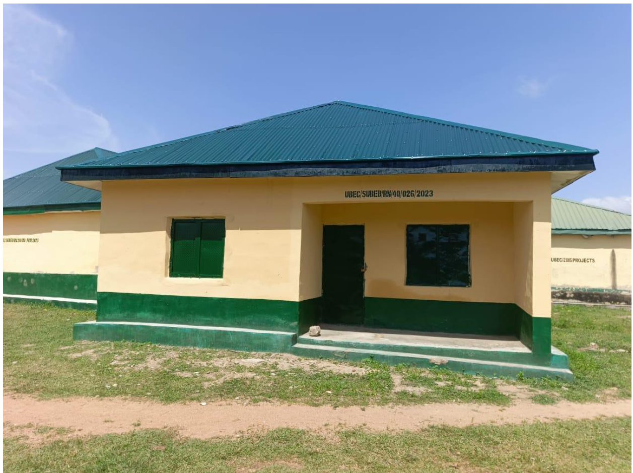
MOH'D NYA PRIMARY SCHOOL JALINGO- BLOCK A, LIBRARY (AFTER
