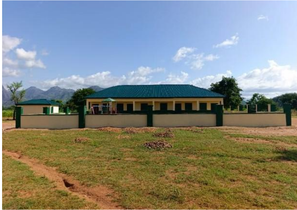
Construction of a block of 2CRMS (ECCDA), at Loro Yakoko P/S
