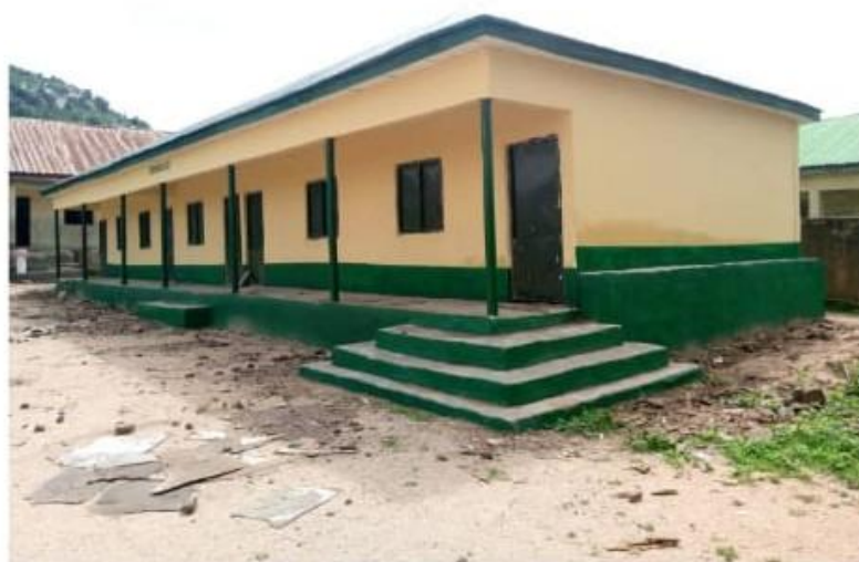
Rehabilitation of 2CRMS, office and store at Gwampo P/S
