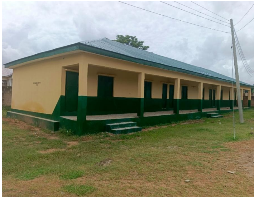
Rehabilitation of 3CRMS, office and store at GJTTS Zing
