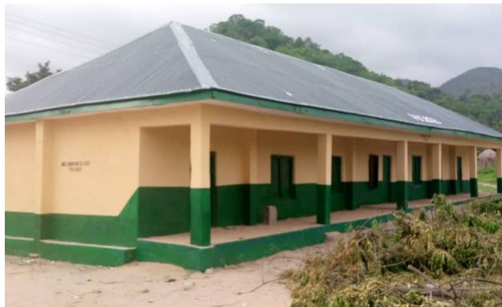
Rehabilitation of 2CRMS, office and store at Nsoreng Gadda P/S
