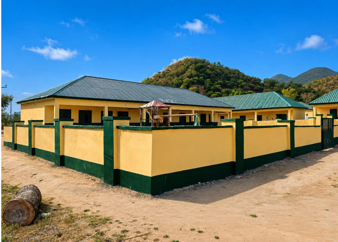
Construction of a block of 2CRMS, office and store at Nsoreng Gadda P/S
