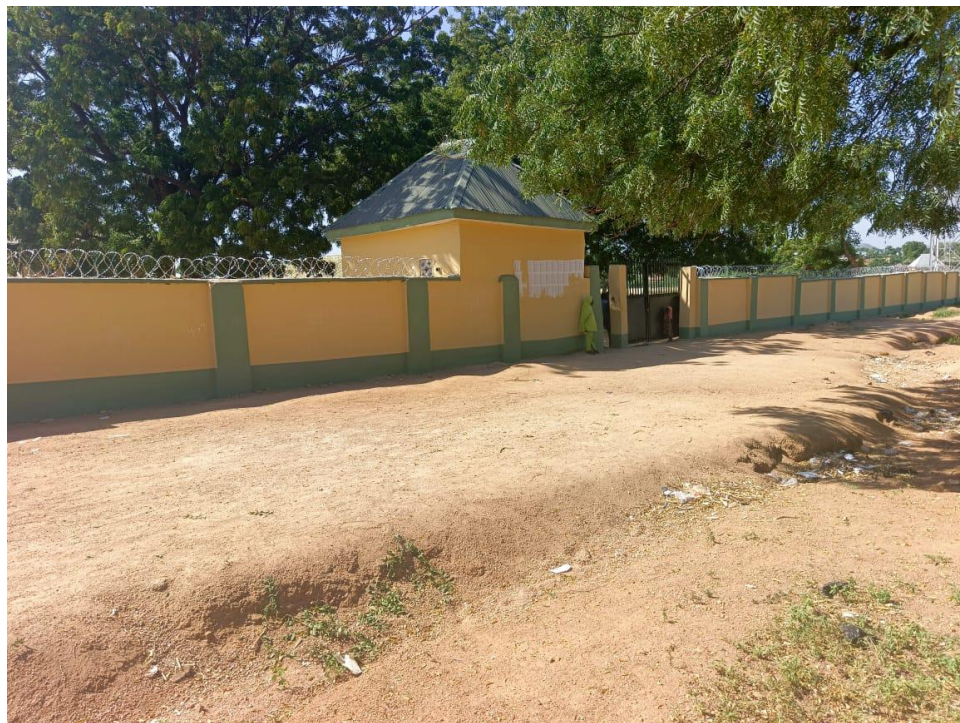
Construction of perimeter fence at Tadova P/S
