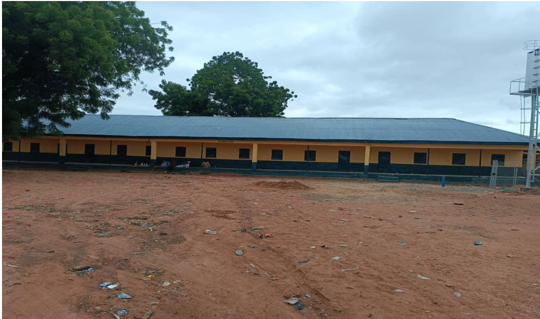
AFTER REHABILITATION, CENTRAL P/S 4C/RM OFF&STR. AT IBI LGA
