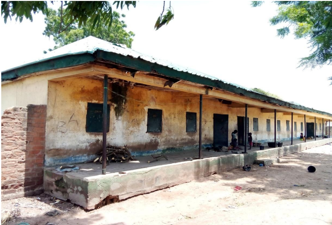
BEFORE REHABILITATION, CENTRAL P/S 4C/RM OFF&STR. AT IBI LGA
